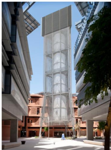
Fig 9: Wind tower in the housing courtyard [13].
